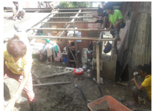
STPB contributed in the food-for-work during the clearing of mudslide and construction of temporary shelter in Ambiong, Baguio City.
